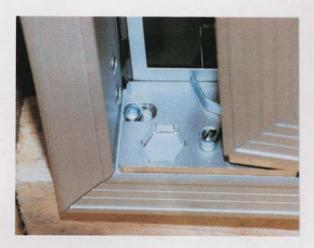
To connect side door, Place hinge pin in next hole to allow more space when connecting.
